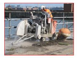
The aggregate in concrete being saw cut was varied, there was limestone, quartz and riverbed gravel.
